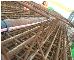
Cable glued inside a penstock
