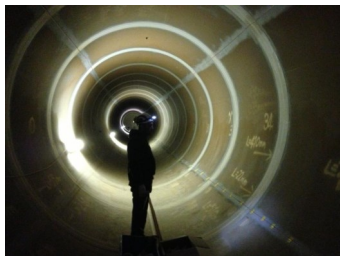
Cable glued inside a penstock
