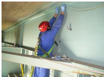
Cable clamped on concrete blocks
